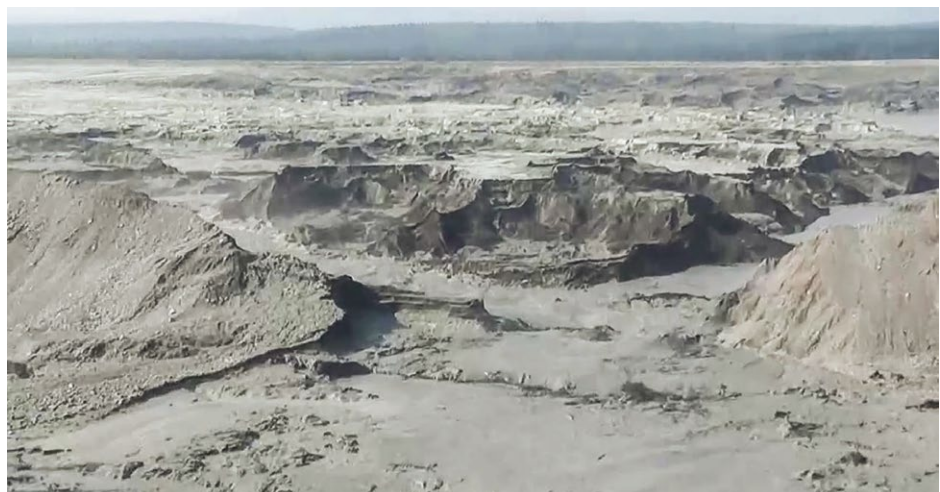
Figure 1: Photo of the Mount Polley Mine Tailings Storage Facility breach, looking upstream.
